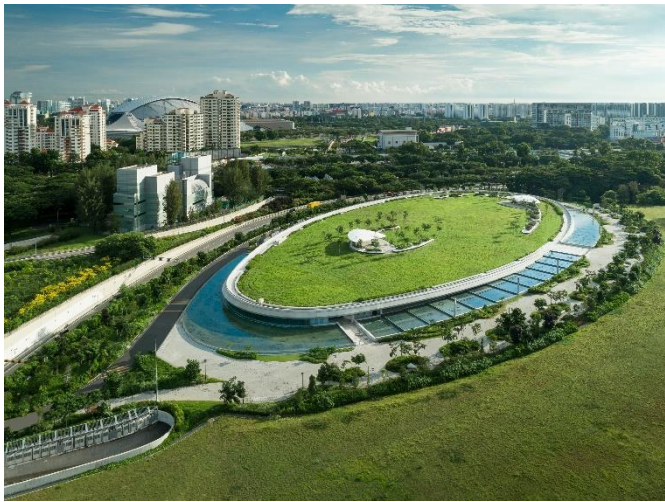
Aerial View of the Keppel Marina East Desalination Plant
